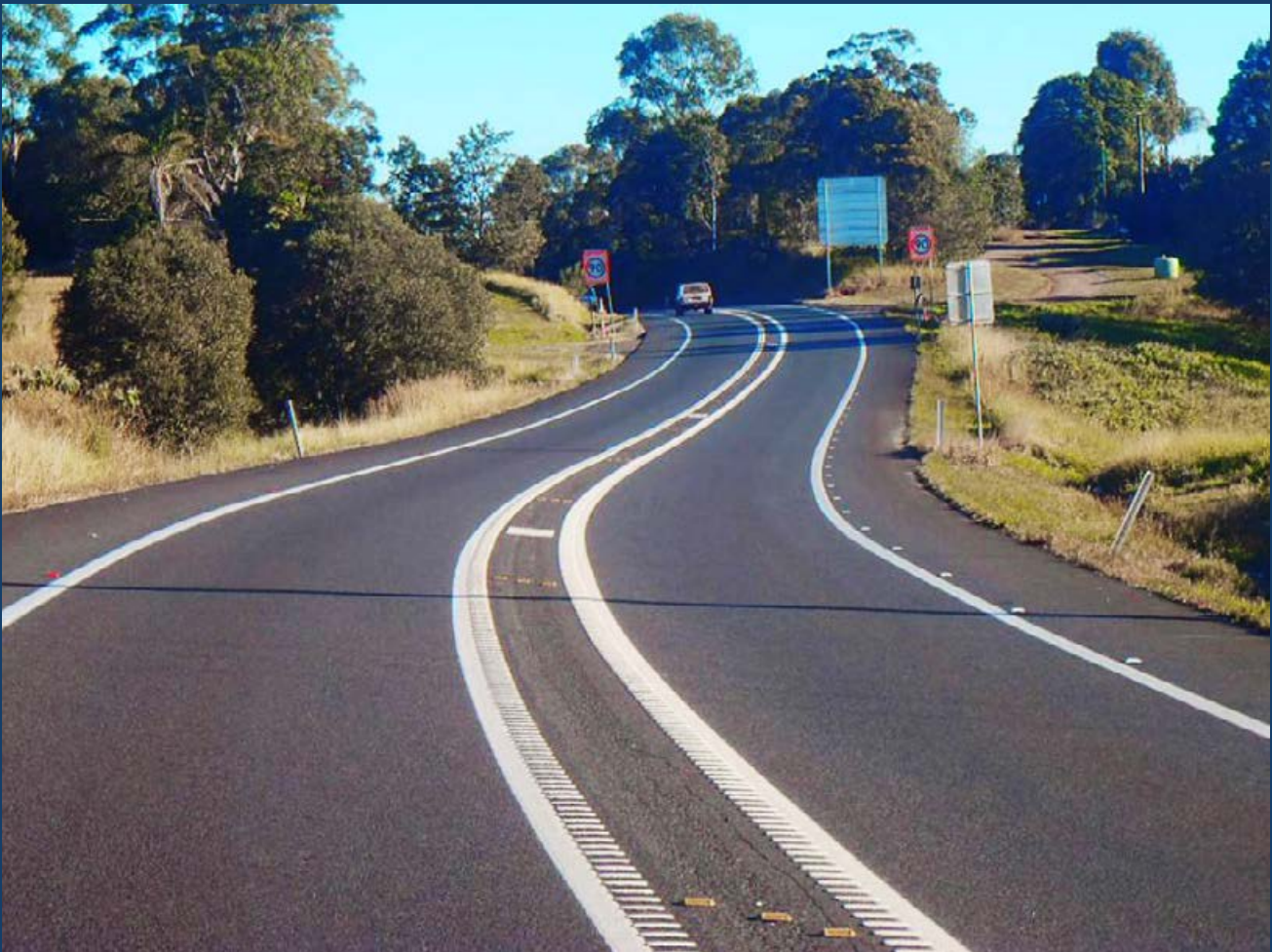
Wide centre line treatments are an effective and relatively low-cost measure to reduce head-on collisions
