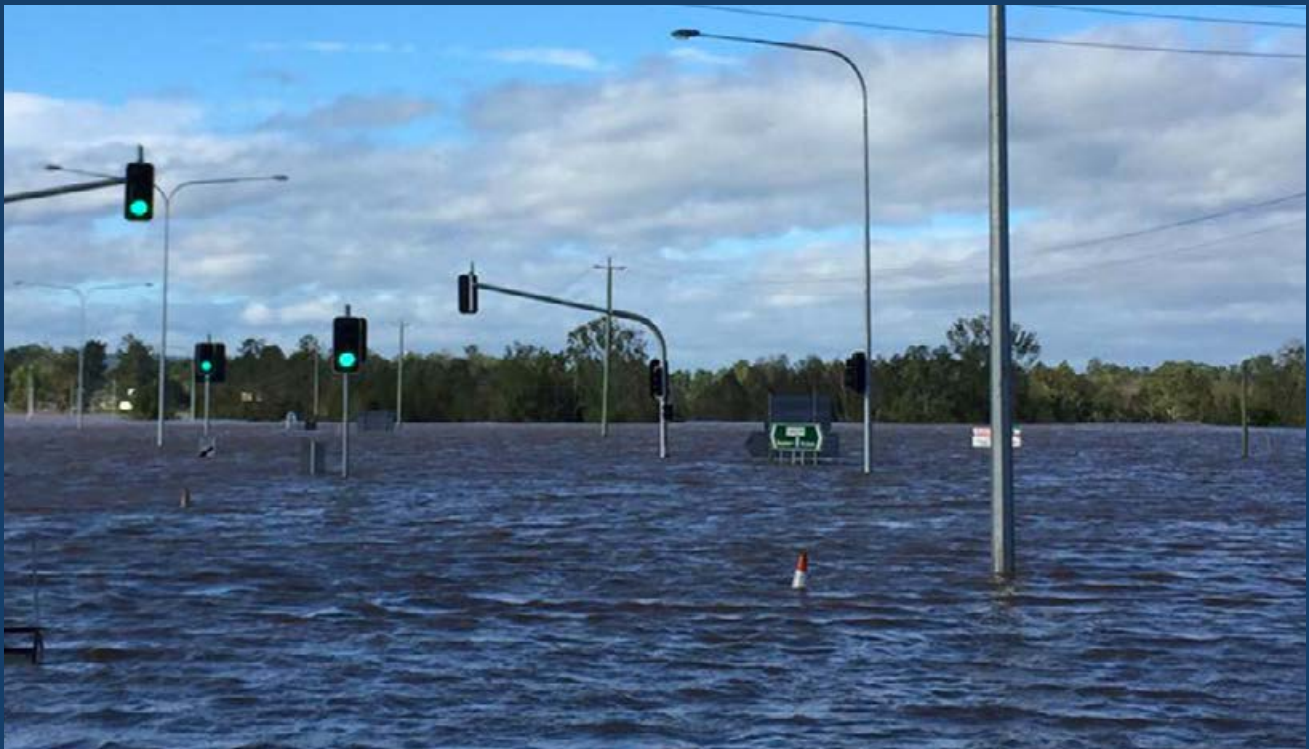
Camp Cable Road, Jimboomba during flooding
