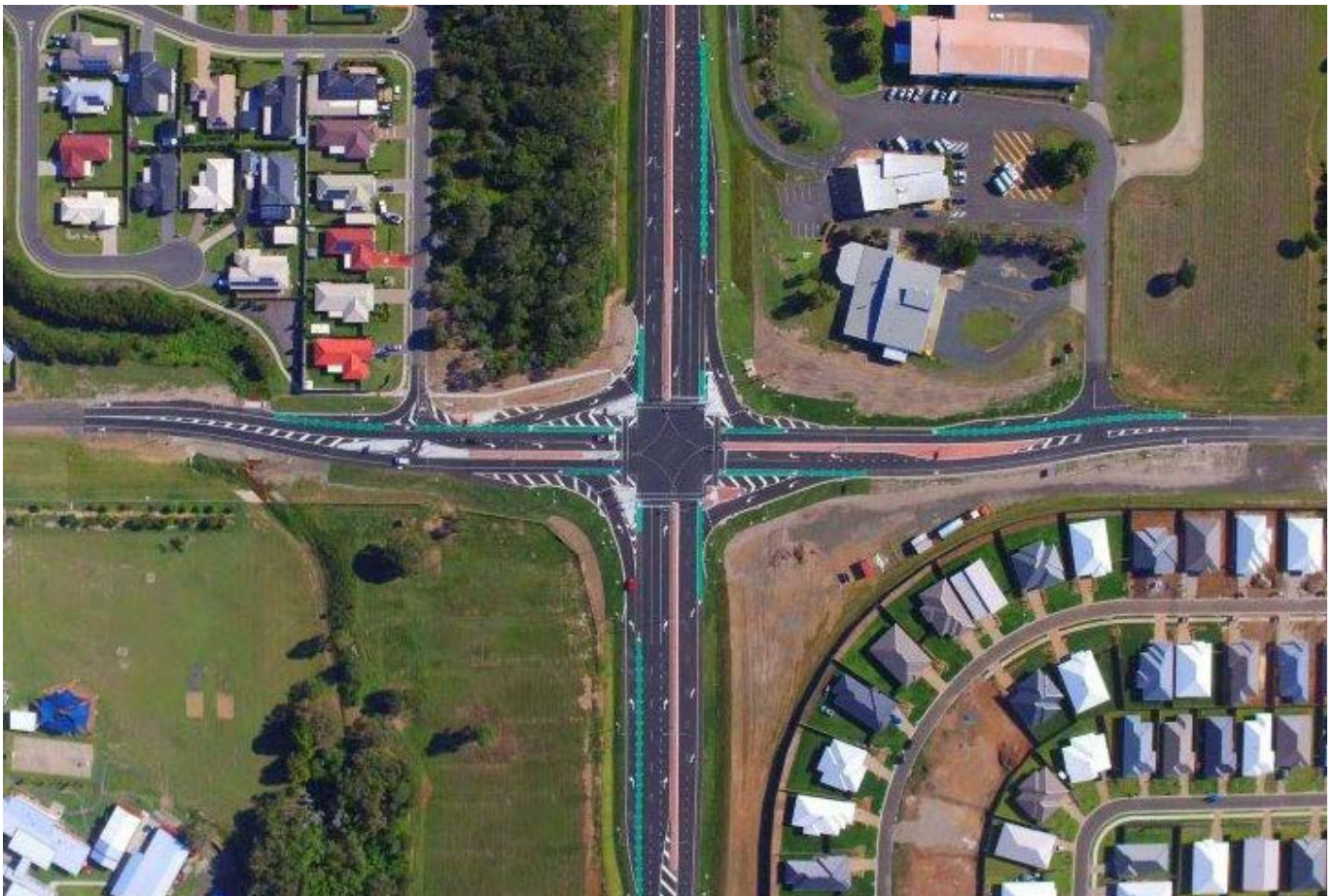
Maryborough–Hervey Bay Road and Urraween Road intersection safety upgrade
