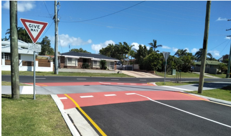
Figure 1.1 – Example of a raised priority crossing for a shared pathway, Mooloolaba Qld
