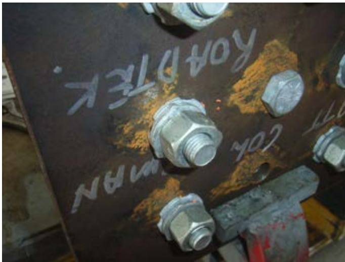
Figure 7.2(c) – Correct orientation for a load indicating washer
