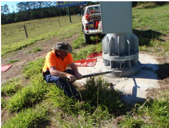
Figure 5 – Extension placed on the end of a ring spanner
