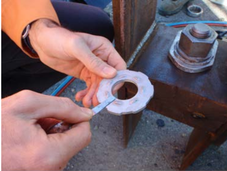
Figure 8.1(b) – How to check a loading indicating washer
