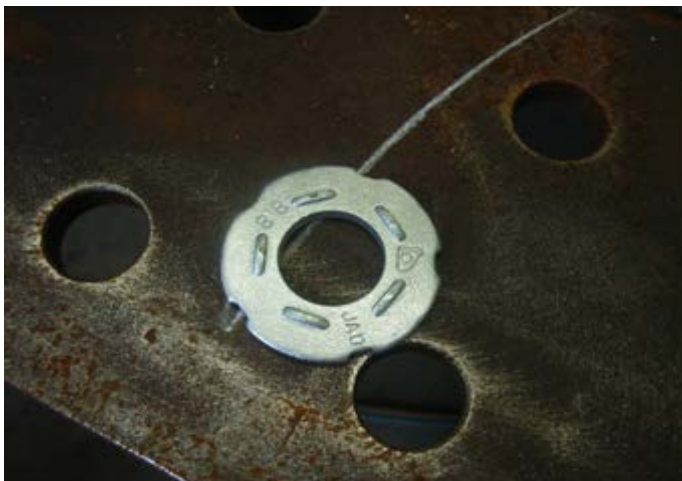
Figure 7.2(c) – Correct orientation for a load indicating washer
