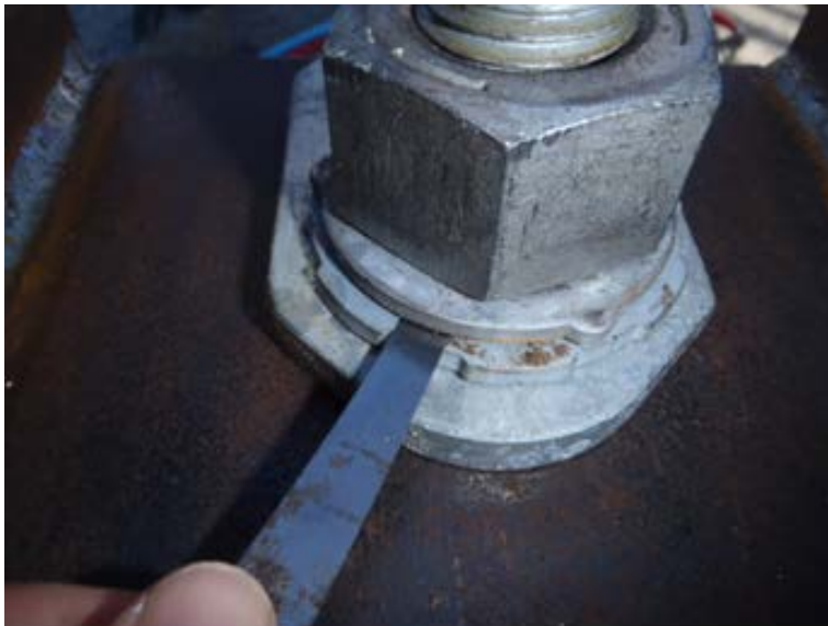
Figure 8.1(b) – How to check a loading indicating washer
