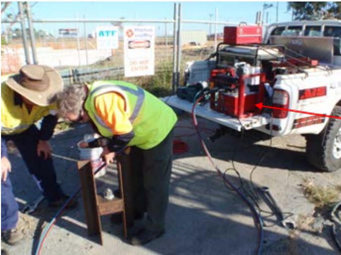
Figure 7.1(b) – Hydraulic torque wrench
