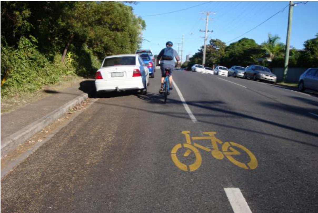
Figure 2.4(b) – Inappropriate application of a Bicycle Awareness Zone in the 'door zone'
