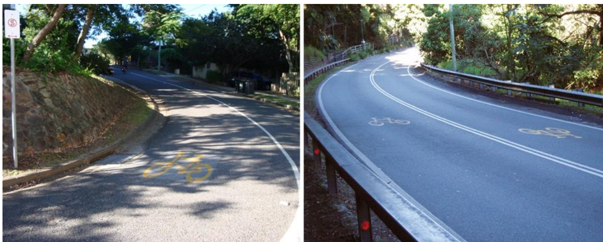
Figure 2.3(g) – Narrow road lanes on sight-restricted corners
