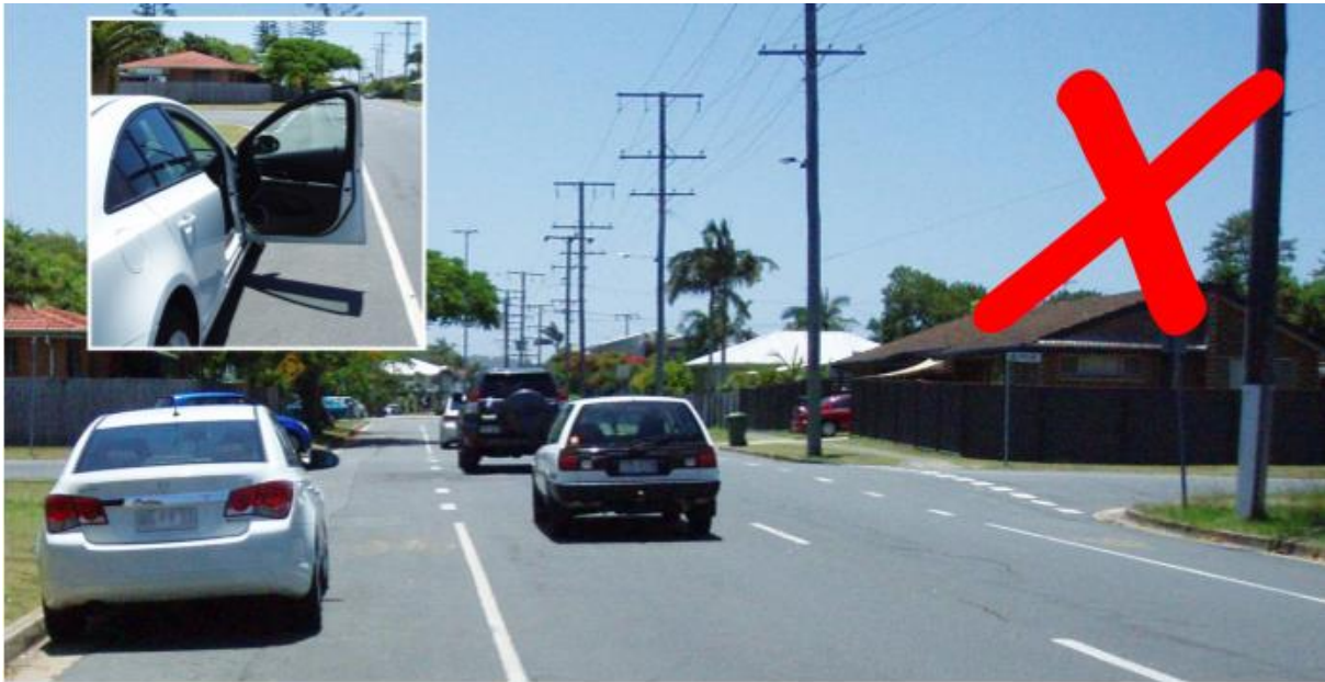
Figure 2.4(a) – Inappropriate use of Bicycle Awareness Zone on the inside of an edge line
