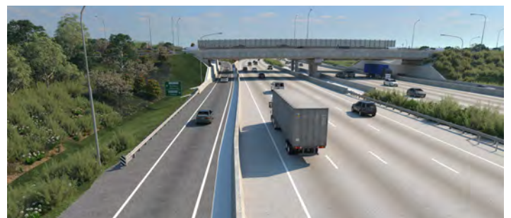
Realigned and lengthened southbound off-ramp.
